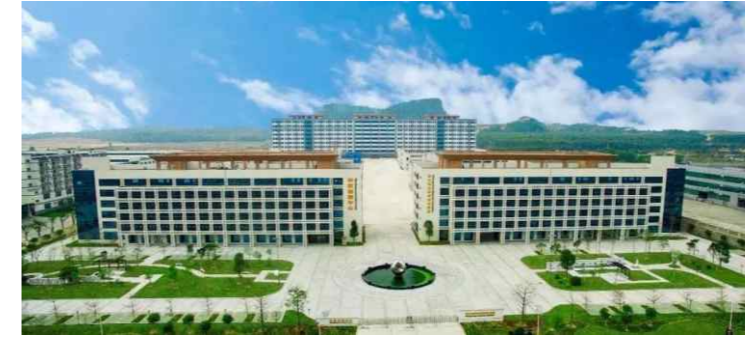
鹤山市人民医院 People's Hospital of Heshan City
